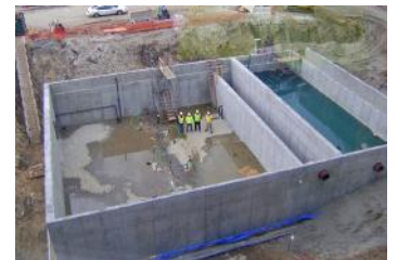
The Wellmark Building in Des Moines constructed this large cistern. The water is collected for irrigation, and supplies 8,000 gallons a day for flushing urinals and toilets. It reduced Wellmark's treated drinking water use by nearly 58%.
